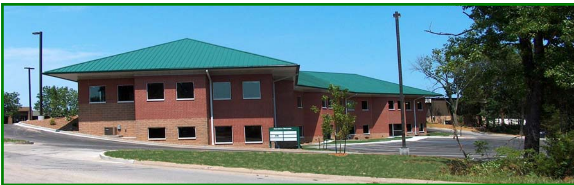
Side View Showing the two story building facing the woods.
